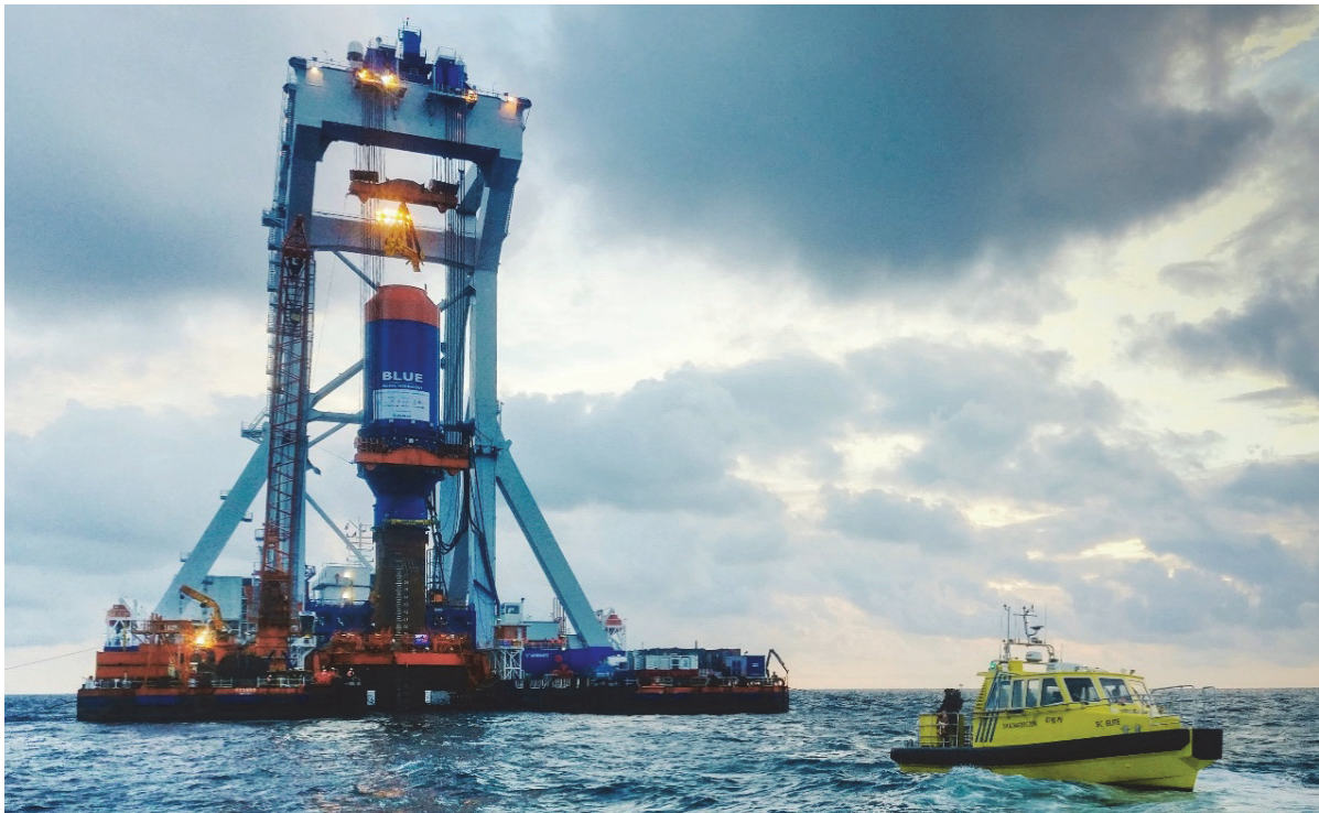
Figure 7. Fistuca's BLUE Hammer deployed on an installation vessel placed on top of a monopile. © Michael Stephenson, The Carbon Trust.
